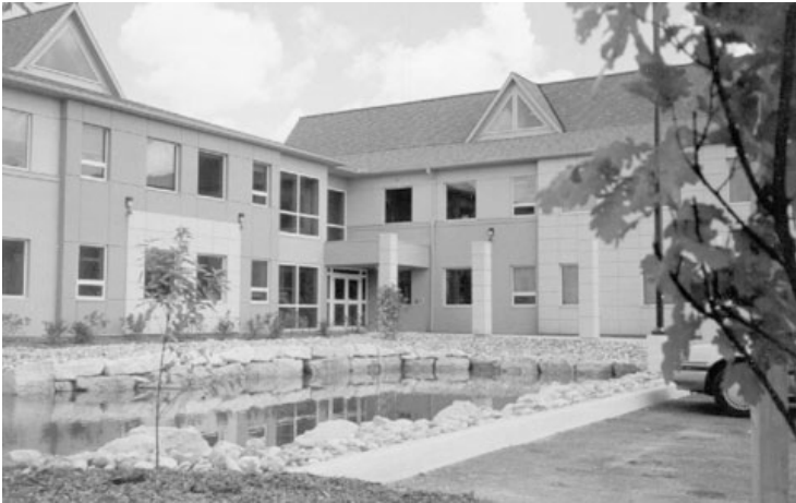
Source: Enermodal Engineering
